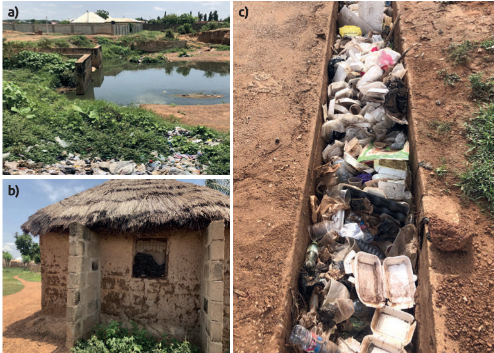
Figure 2: a) A city-level storm drain that stops abruptly in a poor community. b) Piers of concrete blocks added to a mud house to increase its resilience to flooding. c) A roadside storm drain blocked with solid waste rendering it ineffective. (Credit: Ben Howard and Cynthia Awuni)
